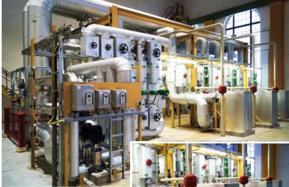
temperature profiles and loads, were considered to insure stable operation at all times. After some adjustments of the parameters – primary temperatures of up to 140°C and secondary temperatures of up to 128°C, with a pressure of up to 22 bar – they had the solution: five units of the brazed plate heat exchanger B649 x 360 with 9 MW each and one unit of B649 x 144 with 4 MW, with 25 bar working pressure.
